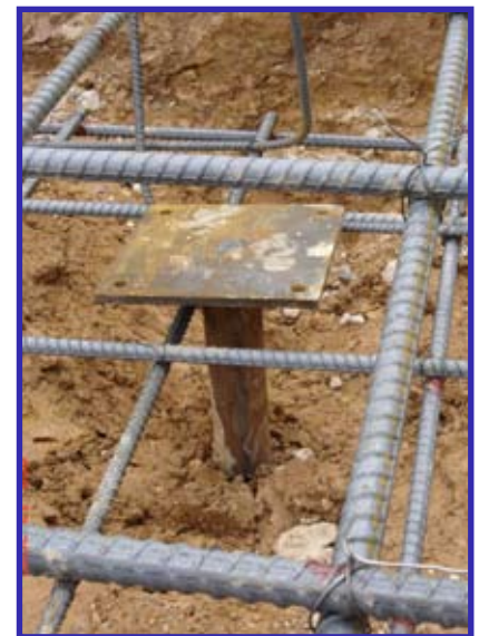
Close-up of Pile with Top Plate
