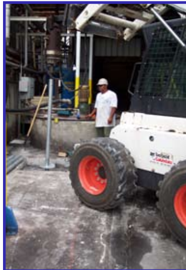
Front and Side Views of Helical Piles Being Driven
