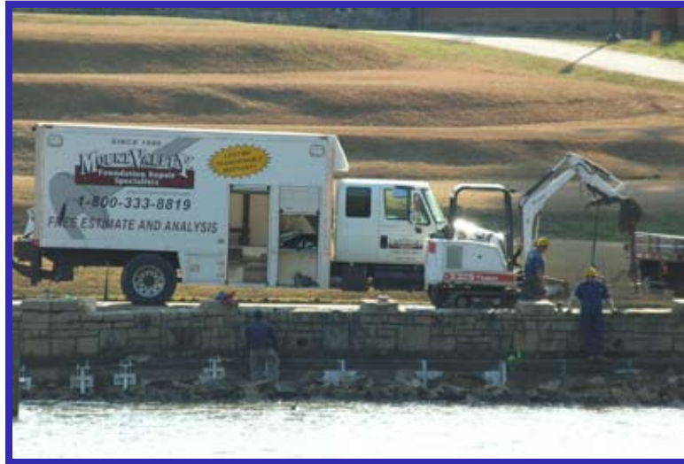
Helical Piles with Lifting Brackets along Retaining Wall
