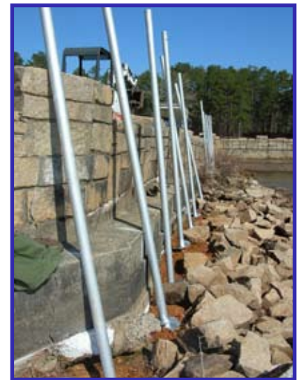
Helical Piles Positioned along Wall
