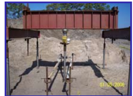
On-Site Pre-Construction Load-Test
