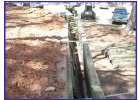
Retaining Wall Under Construction
