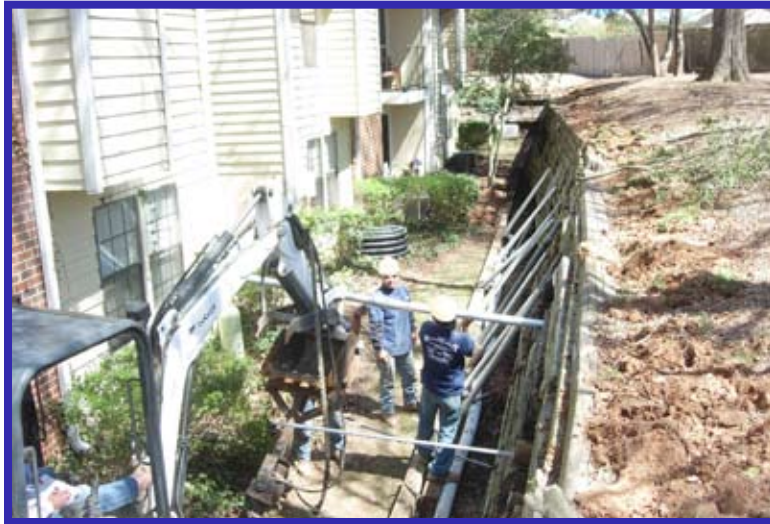
Tieback Helical Piles Being Driven
