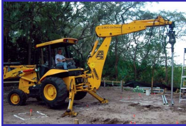
Varying Diameters of Drive Rite Piles Were Used for this Project
