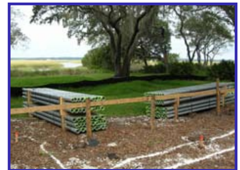
Piles Depths Ranged from 38 to 52 ft size of piers on site.
