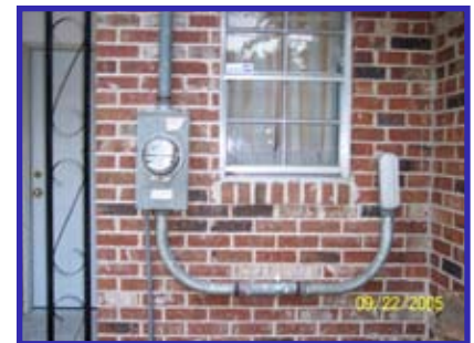
Building Wall - After Repairs
