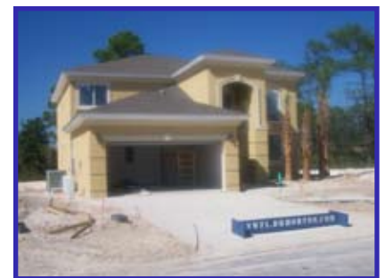
Finished Home with Piles Installed
