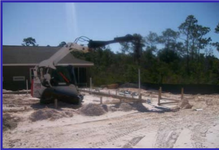
Drive Rite™ 26000 Series Piles Installed Into New Footing
