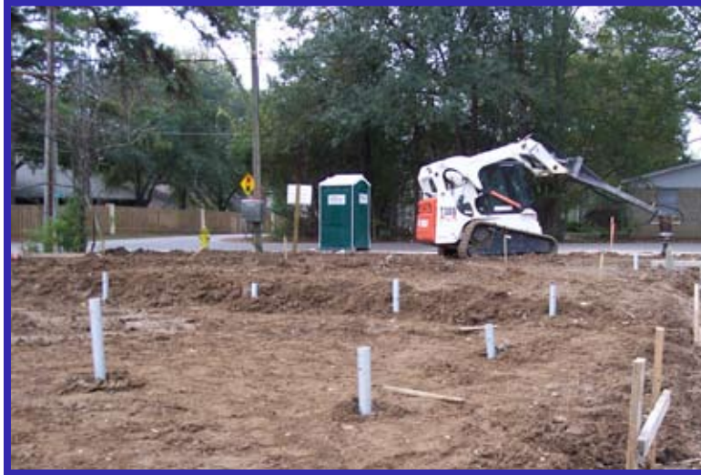
Installation of Drive Rite 26000 Series New Construction Piles
