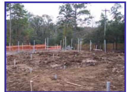
Placement of Helical Piles
