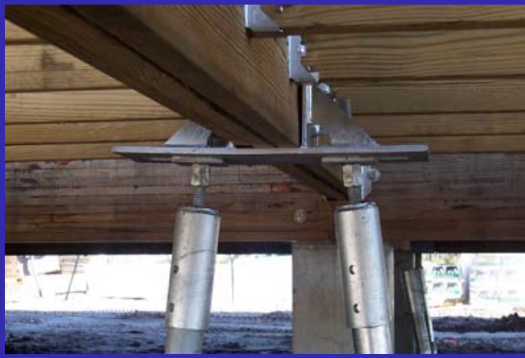
Finished Bracket & Drive Rite Series™ 26000 Series Piles
