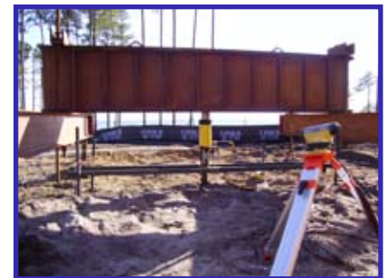
Pre-Installation Load Test
