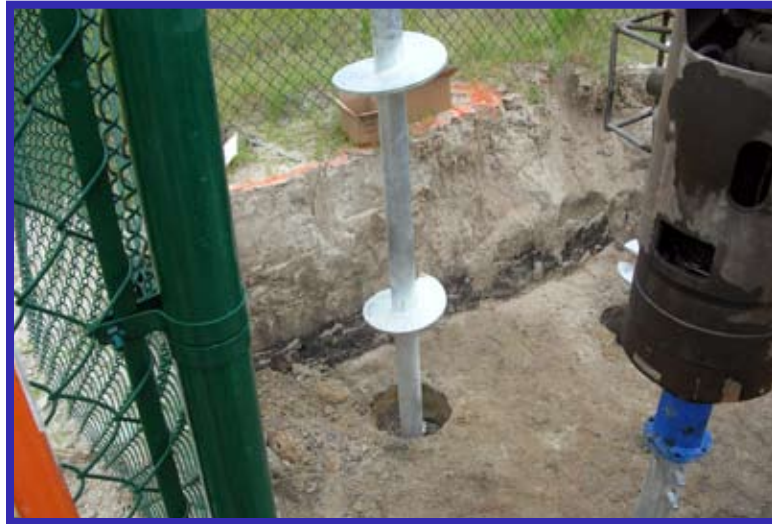
Installation of Drive Rite™ 36000 Series Helical Piles
