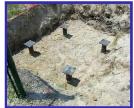
Completed Installation of Drive Rite Piles
