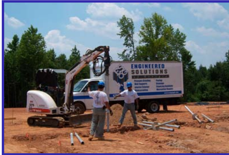
Installation of Drive Rite 25000 and 26000 Series Piles
