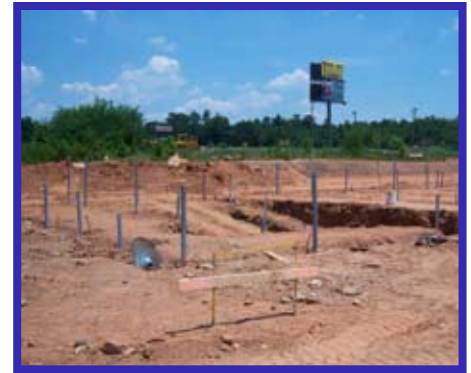
ESOG Installed a Total of 110 Piles
