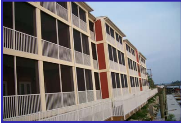
Boardwalk Supported by Drive Rite™ 25000 Series Helical Piles
