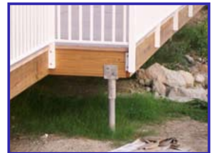
Finished Bracket and Helical Pile
