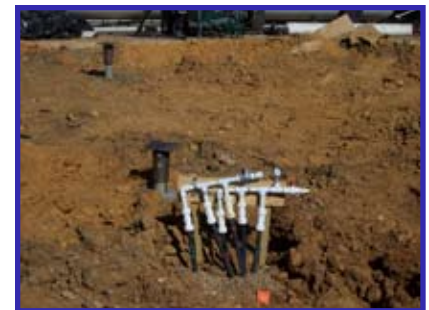
Piles Placed Adjacent to Ground Loop System
