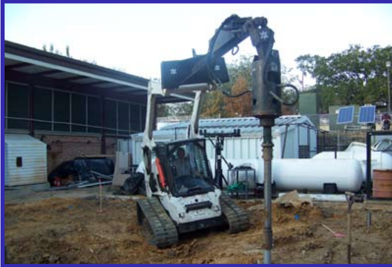
Installation of Drive Rite™ 36000 Series Pile
